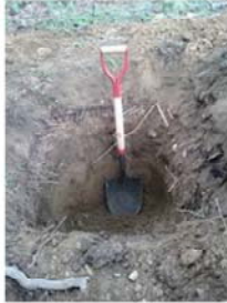
Holes and Shovel
