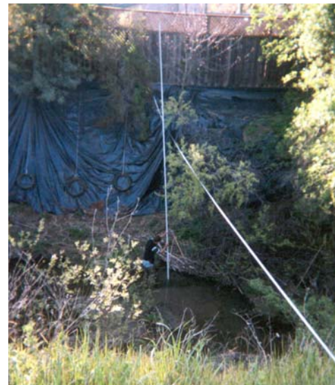
Figure 5. Bank erosion at cross-section 6. 3/19/02.
