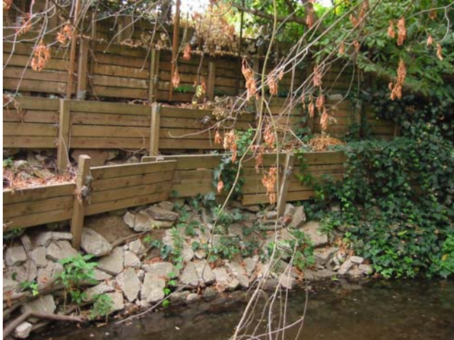
Figure 6. Crib walls and rip-rap near cross-section 8. 10/28/01
