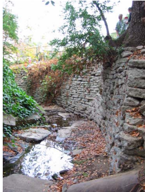
Figure 7. Concrete wall at cross-section 9. 10/28/01.
