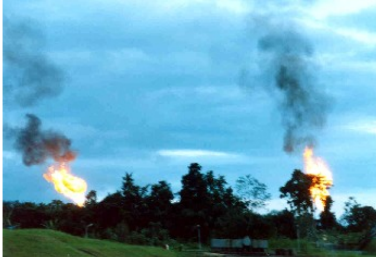
Figure 3. Gas flare of Obama, where a gas scrubber was not equipped
