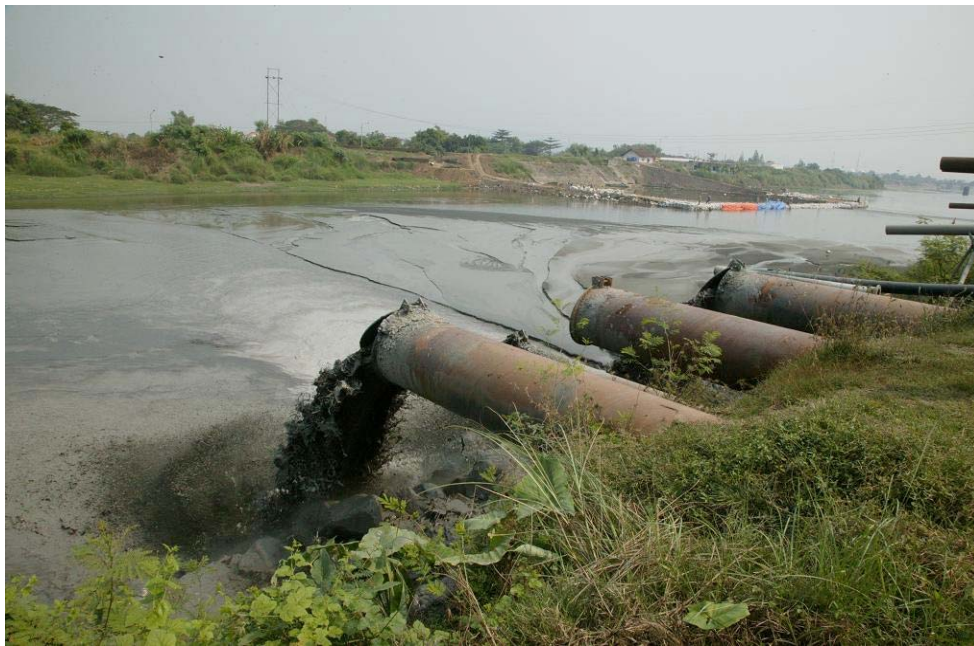
Figure 3. A network of storm drains divert mud from the eruption site into the nearby Porong River to prevent overflow and breakage of the dykes, which keep the mud from further expansion. Photo by Jody Champlin.
