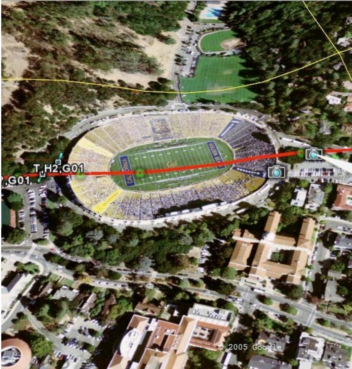
Figure 1: The Hayward Fault (the red line) runs directly underneath UC Berkeley's Memorial Stadium as well as other parts of campus and surrounding areas (Association of Bay Area Governments and U.S. Geological Survey, 2005).
