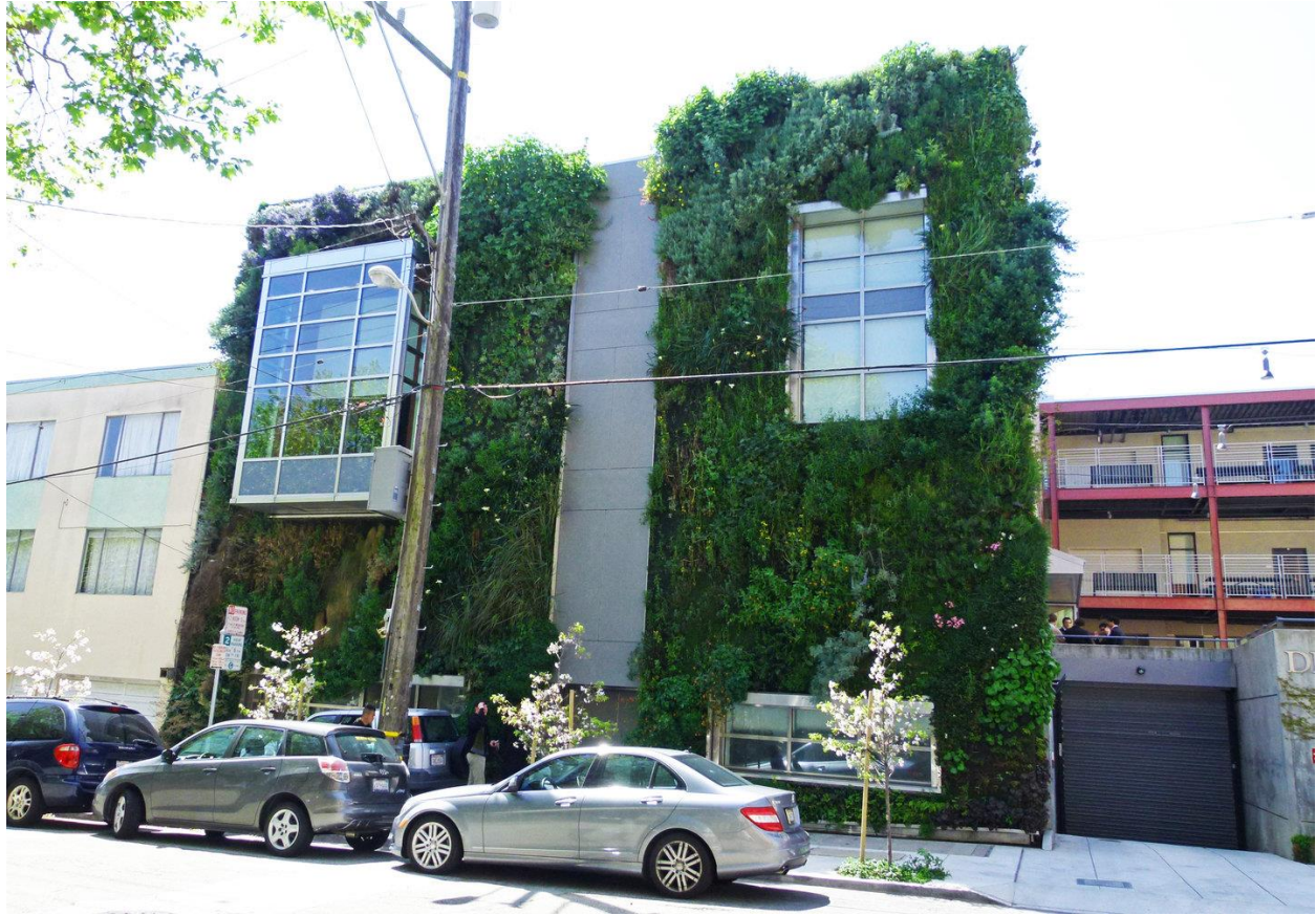
Figure A3: The living wall as seen from Broderick Street. The living wall at Drew makes up the southmost facing wall of the new Sam Cuddeback wing completed in 2011. Although not pictured, there is also a green roof on top of the building. Grey water is filtered through the living wall as to decrease water use.
