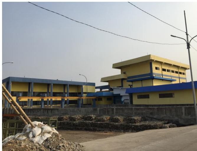
Figure 7: The newest pump house in Pluit that was built as a result of foreign aid from Japan.
