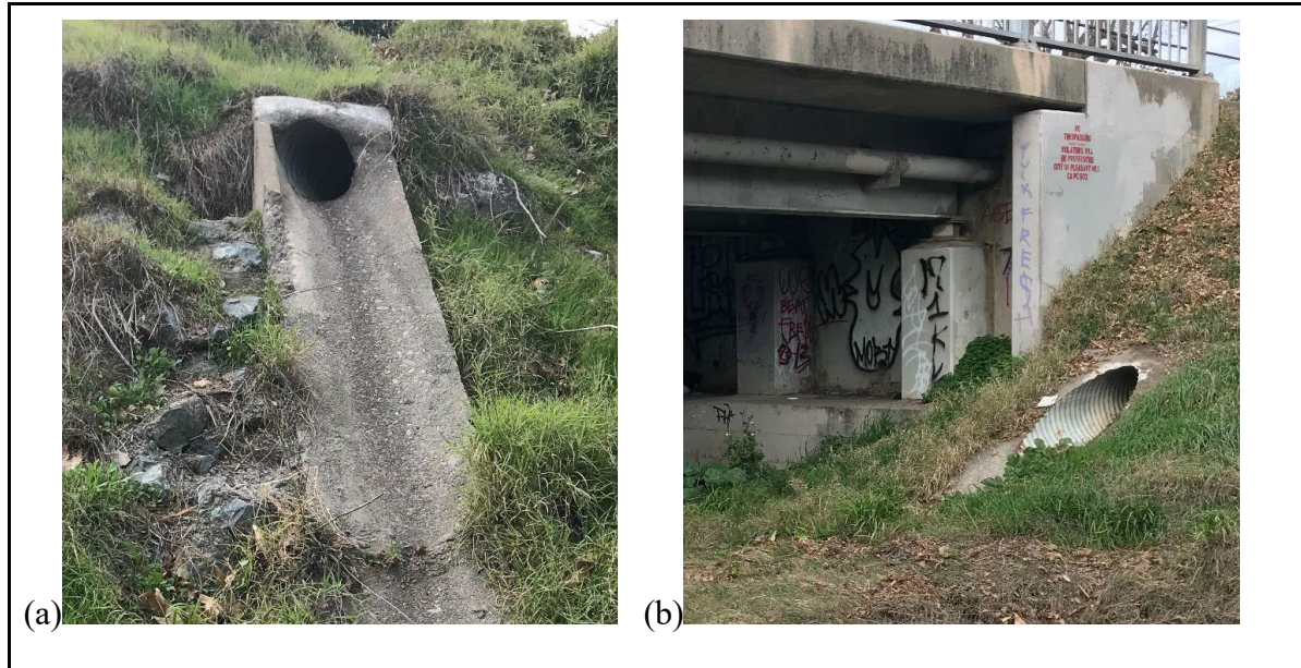
Figure 3. Photos showing the water discharge pipes on each side of the bank of Grayson Creek.
