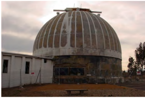
Fig. 6. Telescope destroyed by wildfire at the Mount Stromlo Observatory near Canberra, Australia, on January 18th, 2003. Photo by Scott Stephens.
